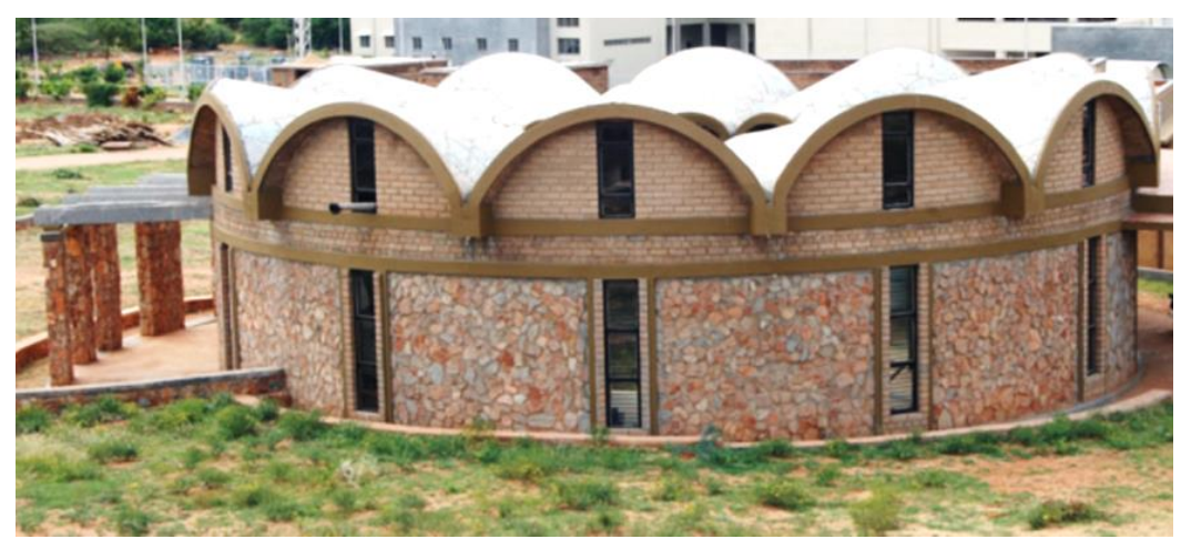
Innovative masonry roofing system at IISc’s exhibition facility at Challakere
